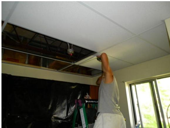
Ceiling replacement at Christensen Courts
